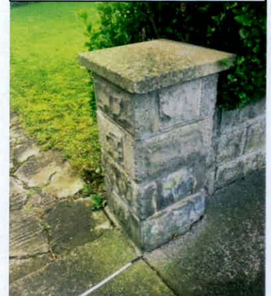
Existing Gate Pier
