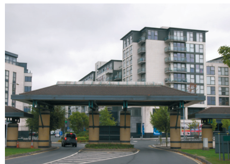
EXISTING 9-10 STOREY BUILDINGS BESIDE TALLAGHT HOSPITAL ENTRANCE & HELIPAD
