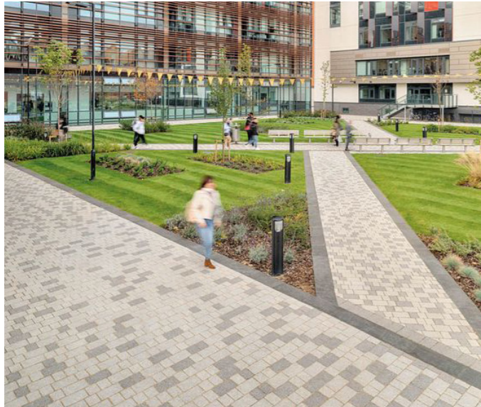
Pedestrian Access - Permeable Concrete Paving
