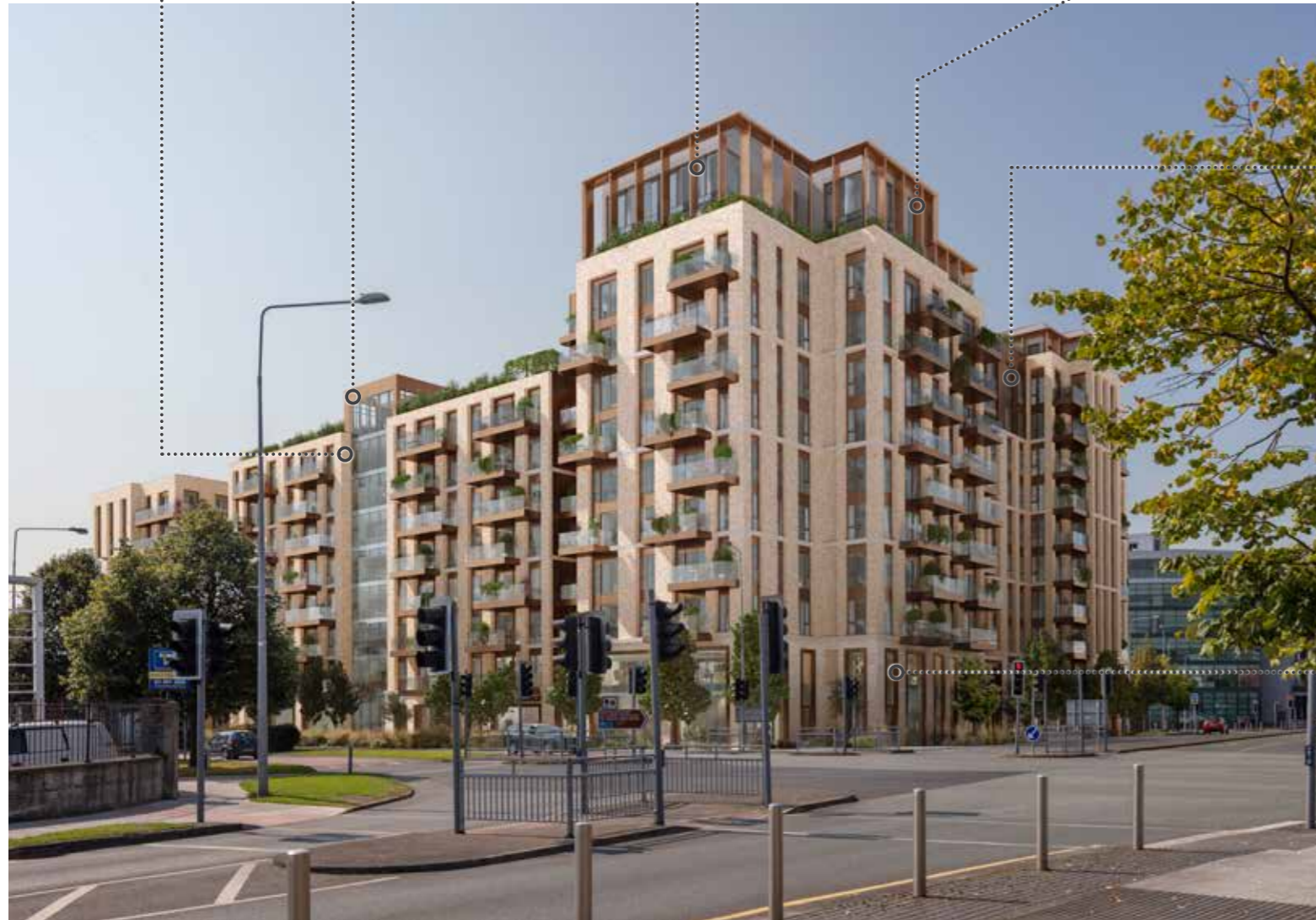
VIEW LOOKING NORTH, AT JUNCTION OF BELGARD ROAD +BLESSINGTON ROAD
