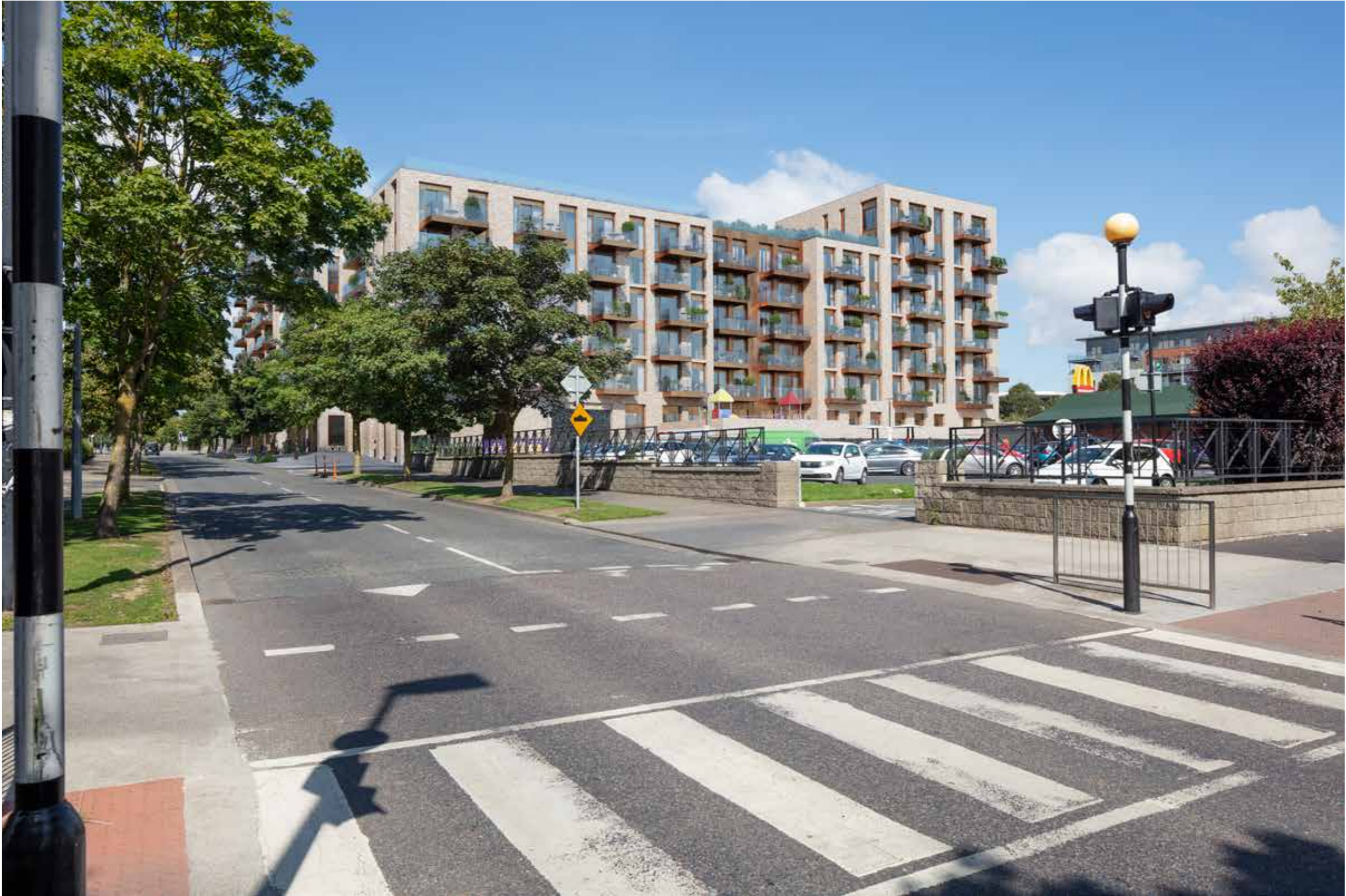
View of southern elevation
