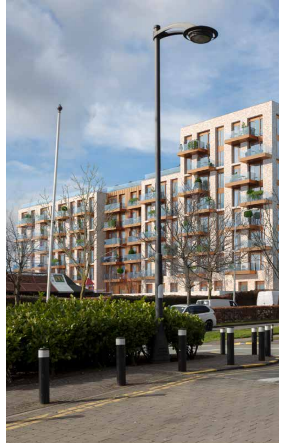
VIEW OF WEST FACING ELEVATION
