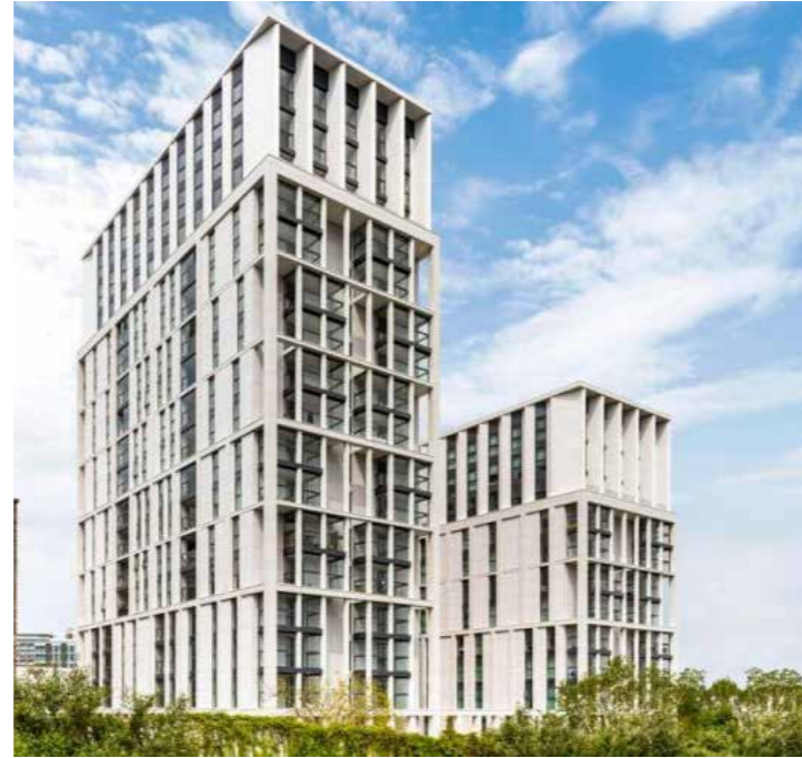
FEATURE CORNER SITE BUILDING WITH LIGHTHOUSE FEILDEN CLEGG BRADLEY - BATTERSEA EXCHANGE
