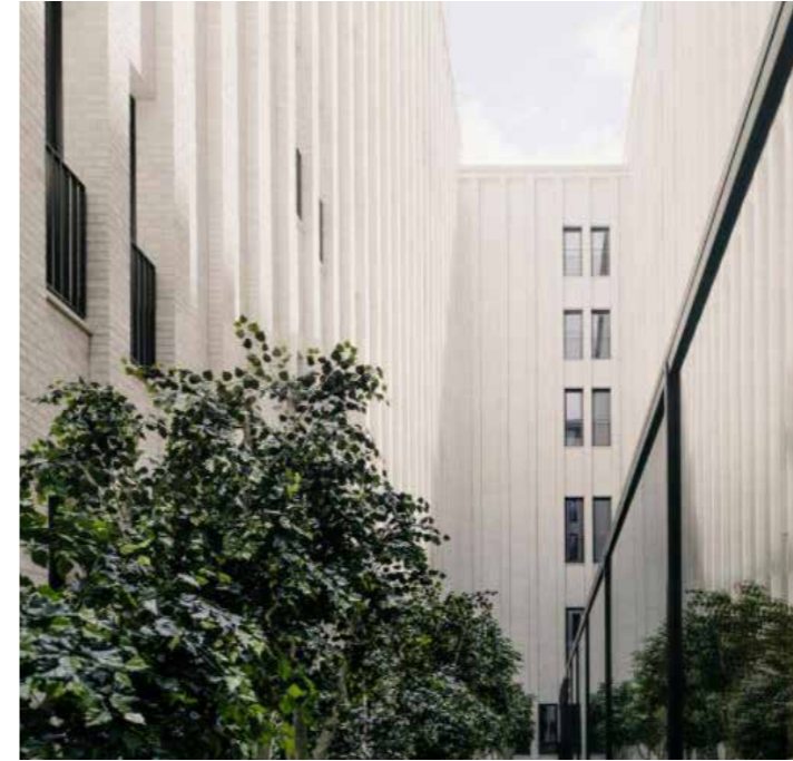
BRICK DETAILING TO COURTYARD DAVID CHIPPERFIELD ARCHITECTS - ONE KENSINGTON GARDENS
