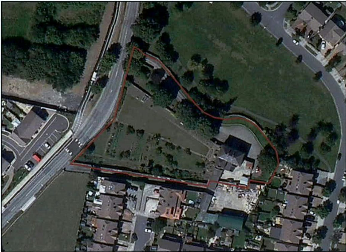
Plate 1 Aerial image of proposed development site at Prospect House showing an overview of the walled garden to the west of the house and the segregated yard and outbuildings at the rear of the house (OSi Licence EN 0077922).
