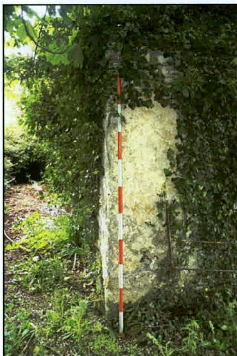
Plate 19 Northwest corner of gate lodge (view to SE).
