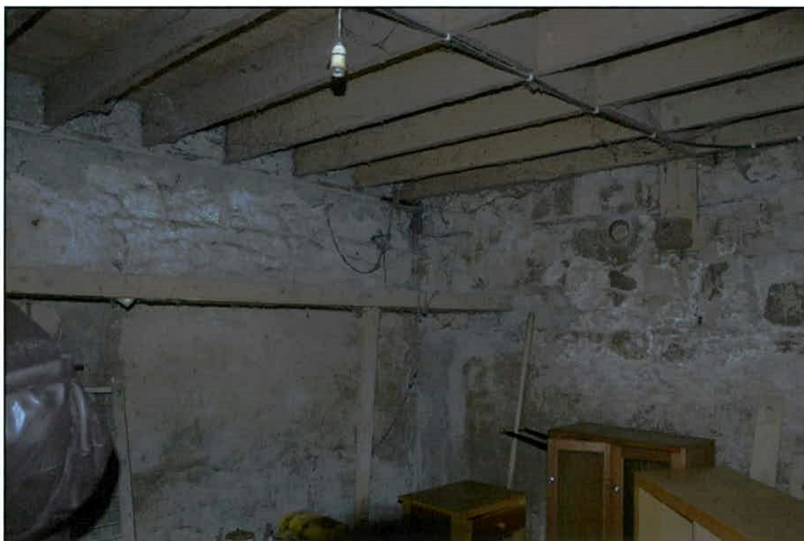
Plate 8 Downstairs interior of southernmost stable (view to SW).
