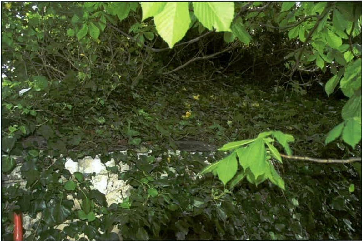
Plate 20 Roof of gate lodge beneath cover of ivy (view to SE).
