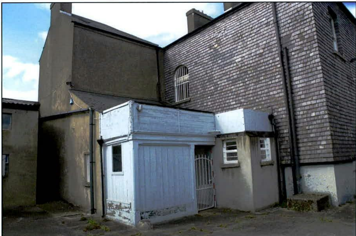
Plate 3 Back porch surmounted by water tank (view to NNW).
