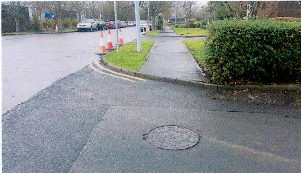
Existing Estate typical footpath kerb at accesses (source: SRC)
