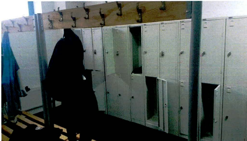
Existing Locker/Changing Room in HQ building (source: SRC)
