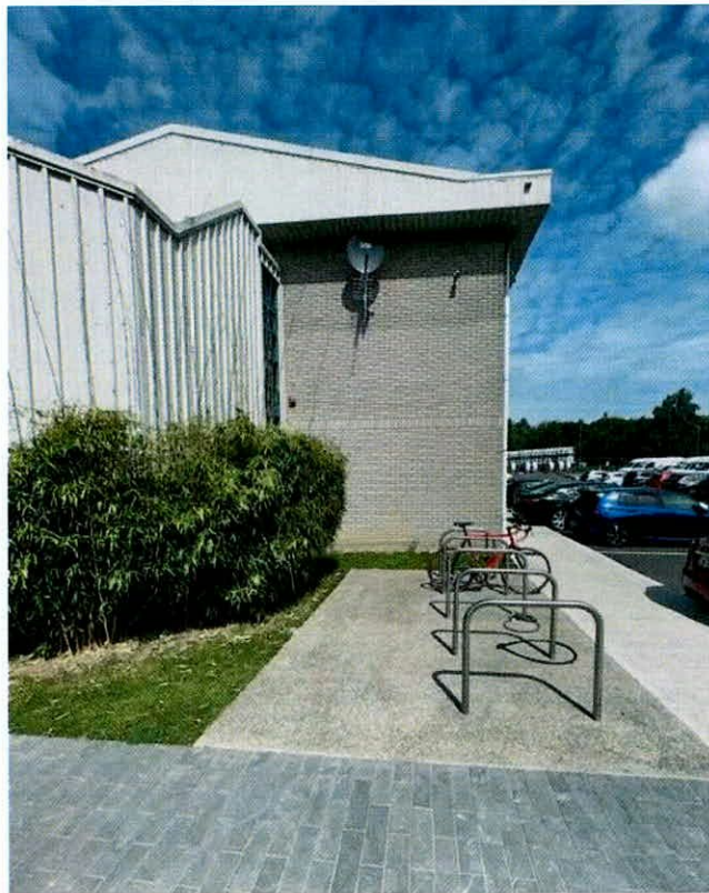
Fig. 1 - Existing Bicycle Parking
