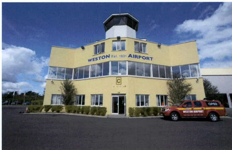
Figure 3.2. Weston Airport (Viewing South - East)
