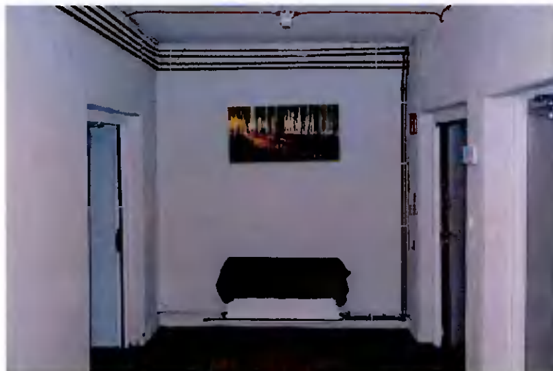
Plate 35: View to north in basement hallway
