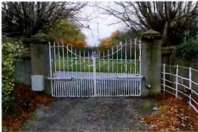
Plate 12: Interior face of gates
