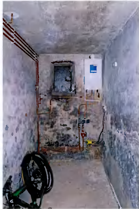
Plate 40: View to east in boiler room
