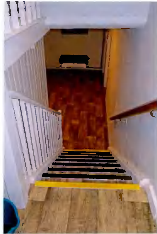
Plate 32: View of staircase from mezzanine
