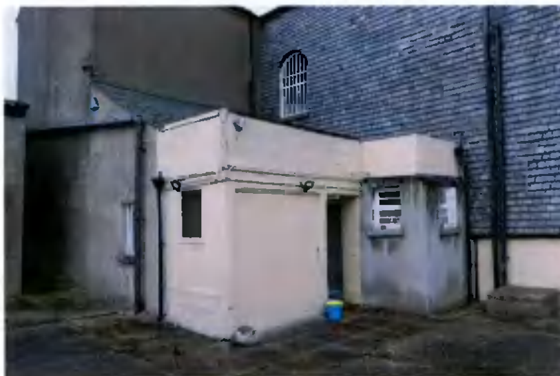
Plate 4: Structures at the rear of the house
