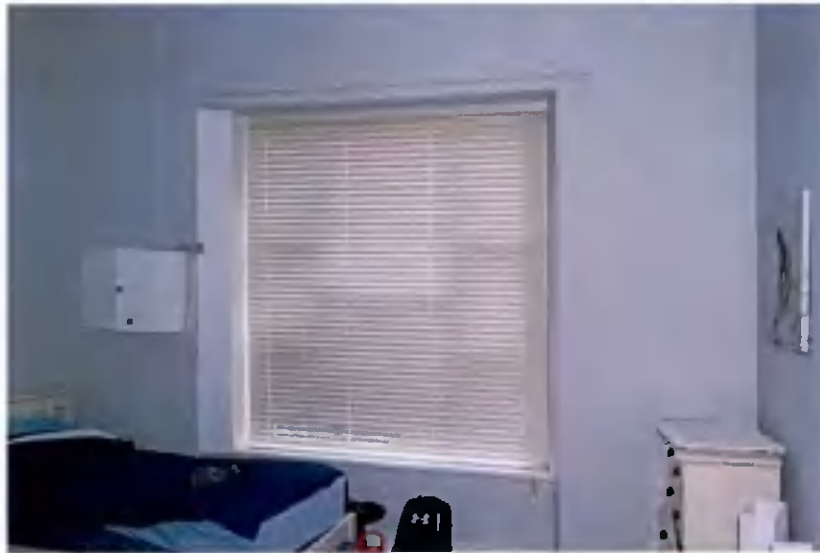
Plate 26: Window in rear bedroom on ground floor
