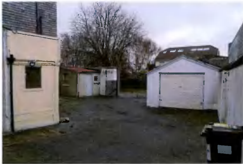
Plate 5: View eastward in the yard
