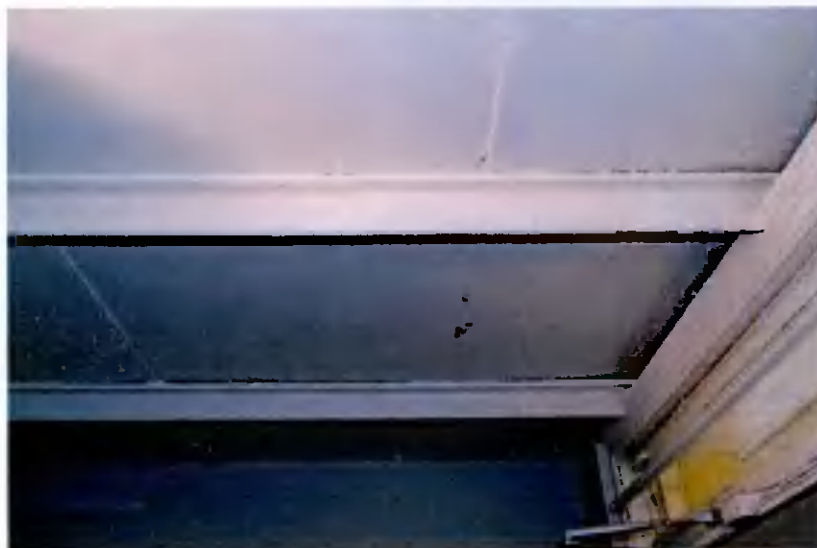
Plate 31: Ceiling in utility room
