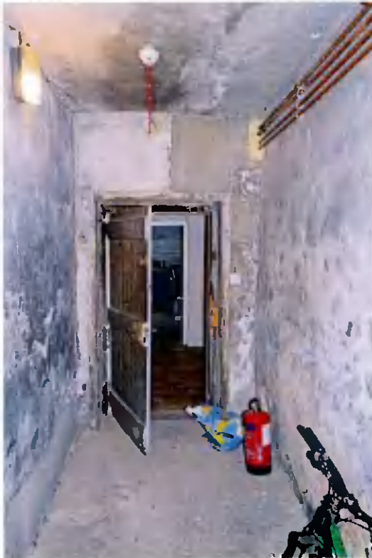
Plate 41: View to west in boiler room
