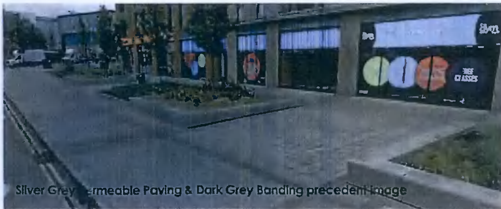
Fig. 27: Poor quality external environment precedent image on p. 22 of the Design Statement
