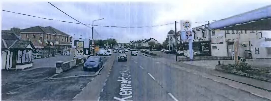
Fig. 19: Existing 2 storey height of shopping centre relative to the existing public house
