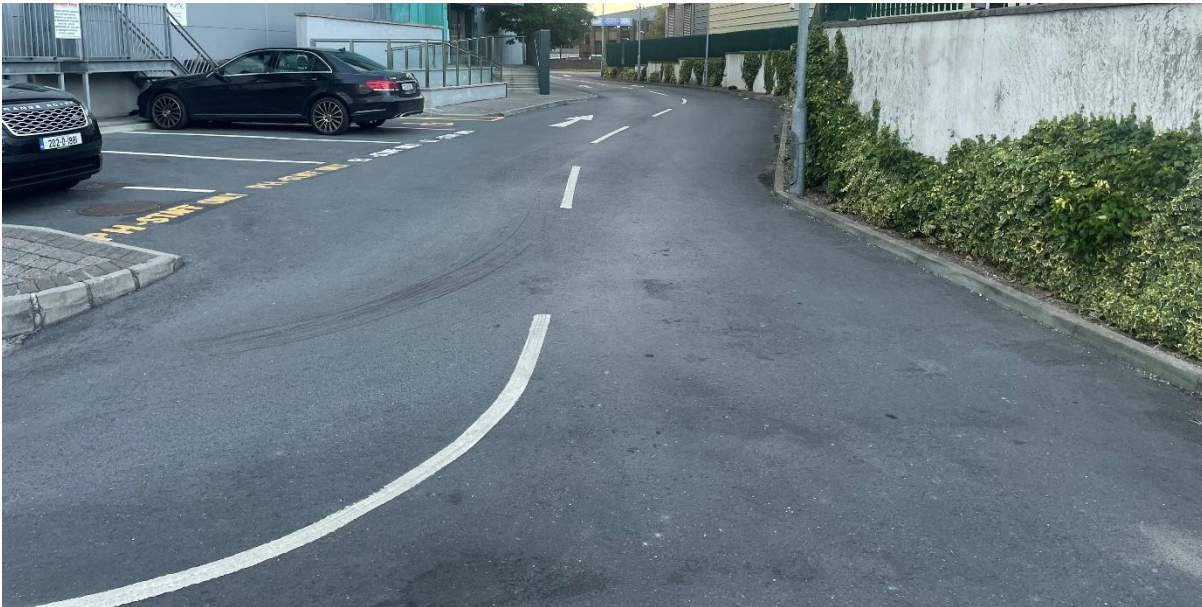
Figure 2 Looking north along the existing access road
