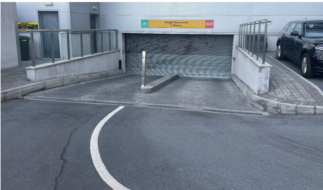
Figure 4 Ramp down to existing carpark
