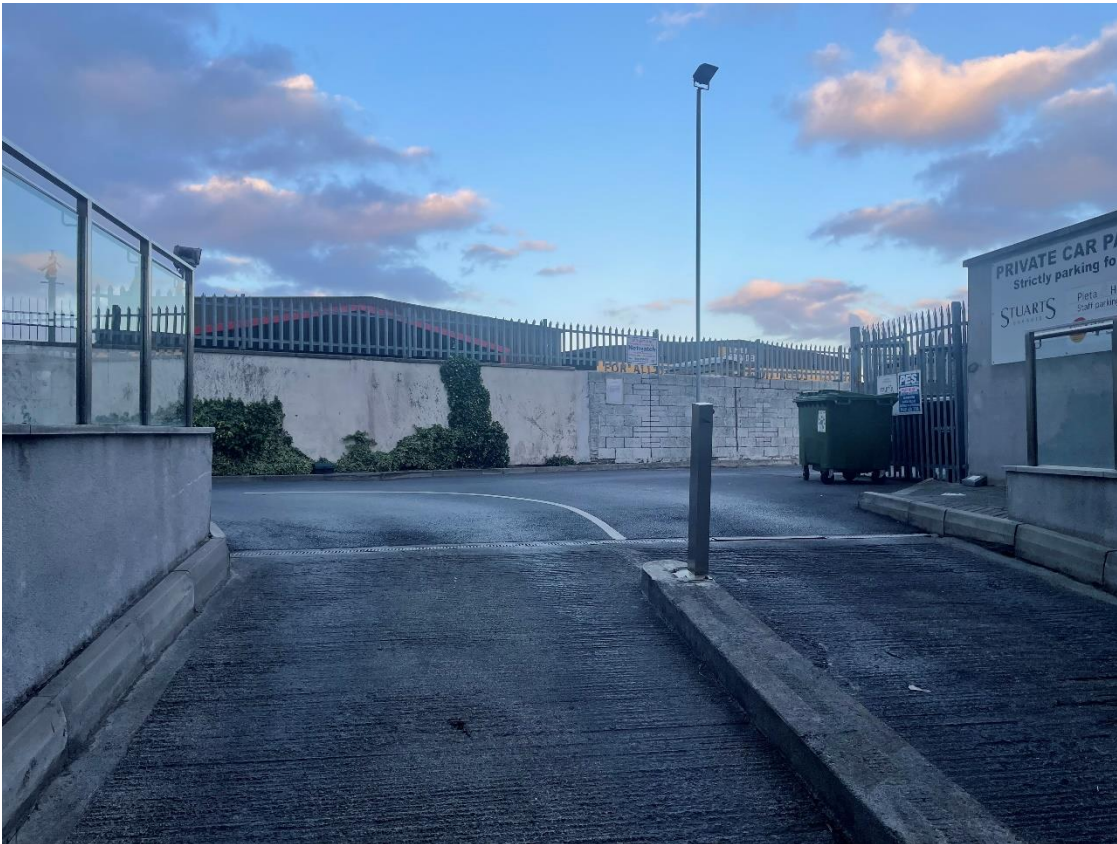
Figure 5 Ramp up from existing carpark
