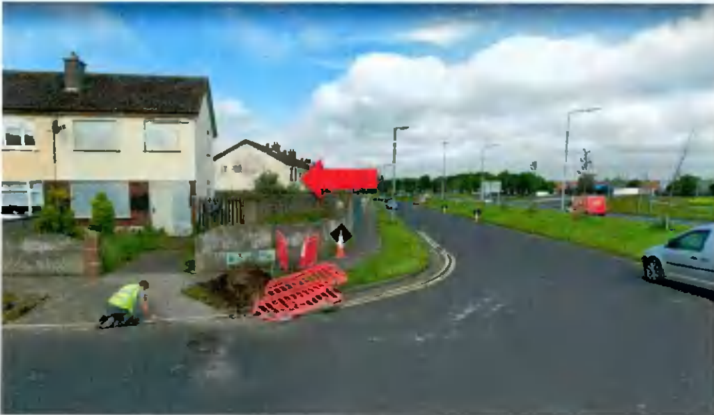
No. 2 Glenfield Drive – opposite the proposed development. (Not Built Yet) Successful example of a corner house, which breaks the established building line.
