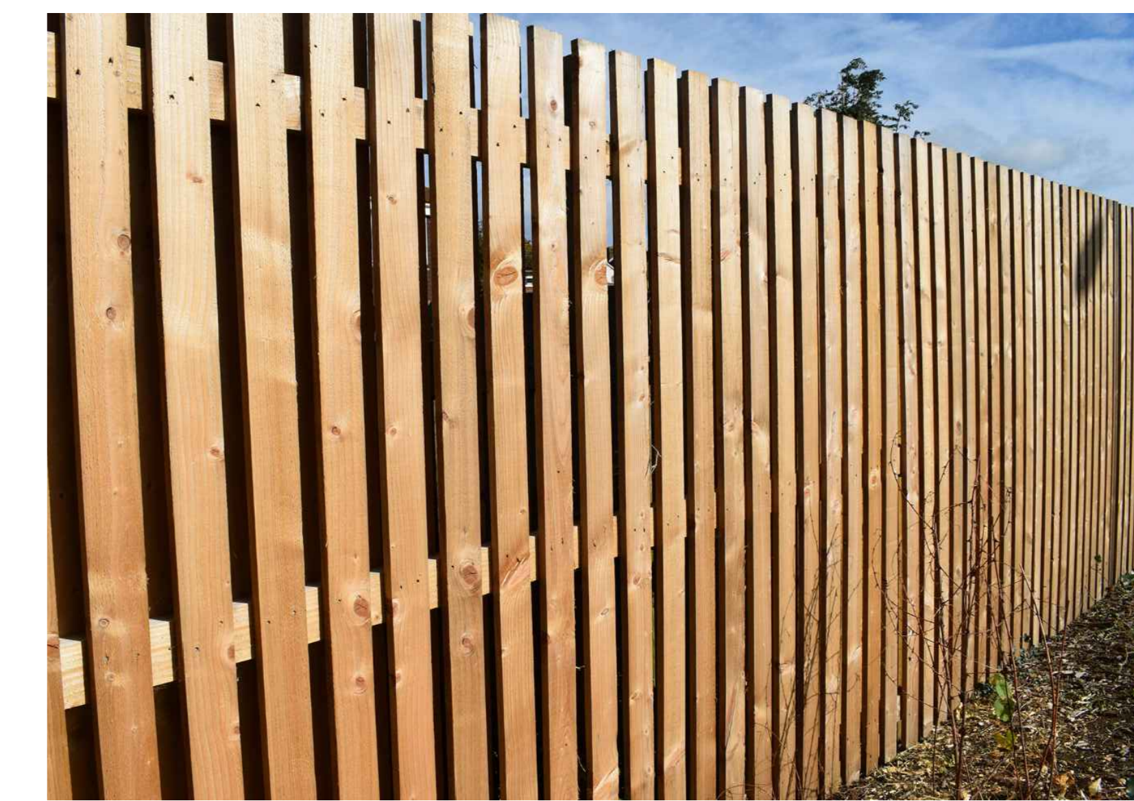
VIEW OF TYPICAL SCREENING NTS
