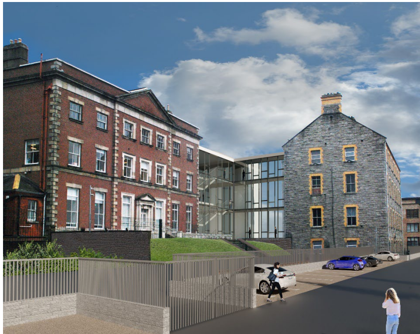
Fig. Illustrative only – not reflecting the planning application detail – please refer to drawings
