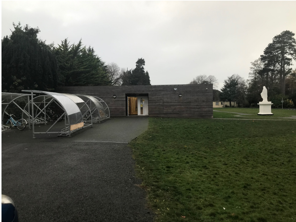
Plate 4. Temporary school building, from east.
