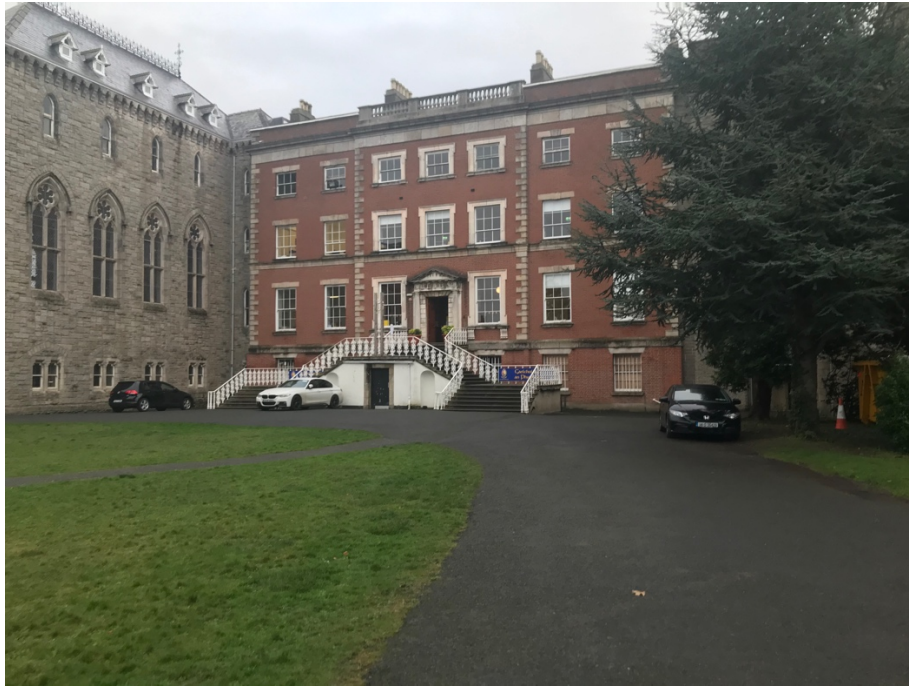
Plate 2. Front elevation of 1732 mansion.
