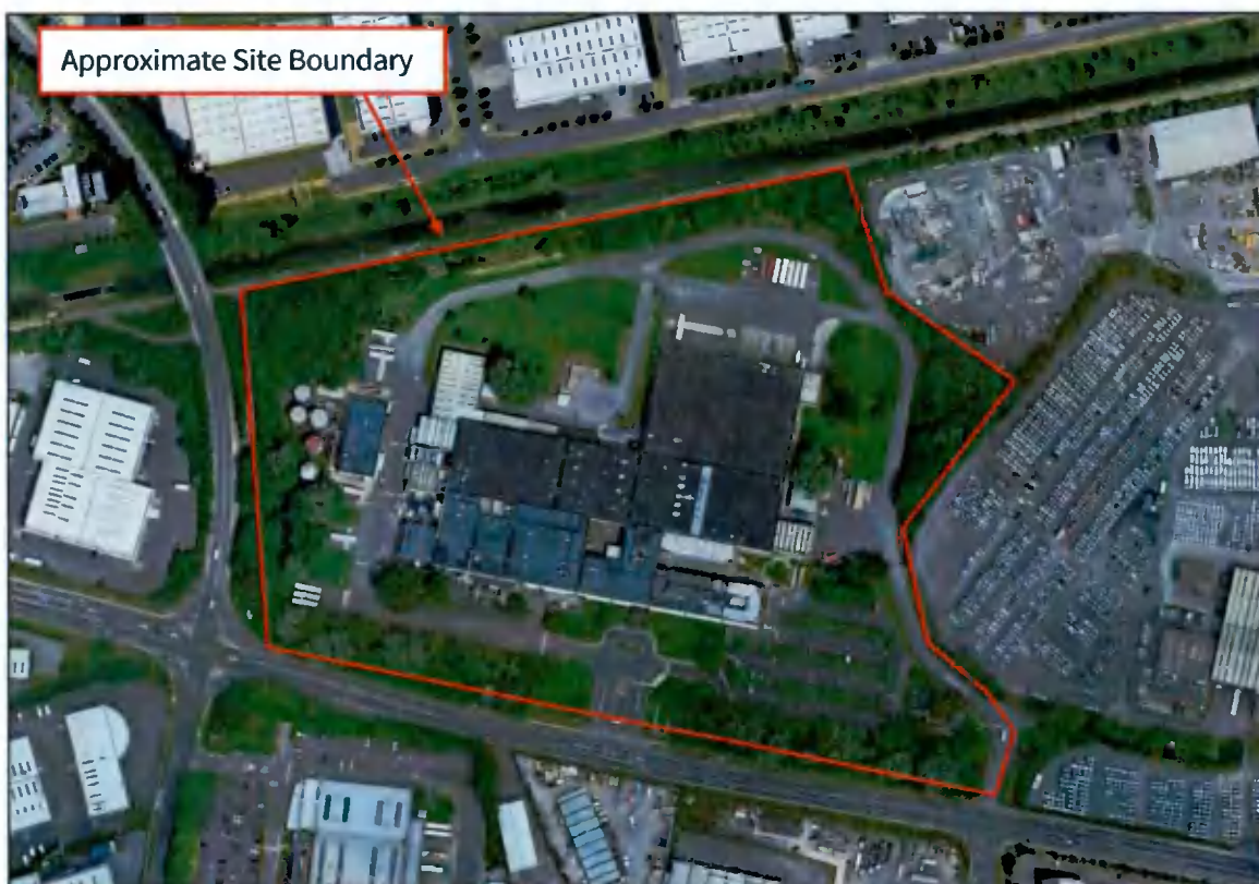
Figure 2.1: Site Location (Google Maps, 2020)
