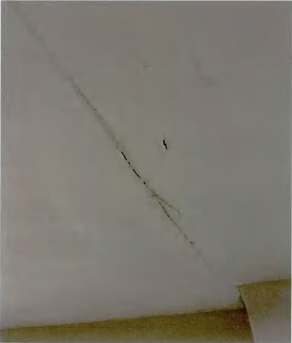
Leaking roof
