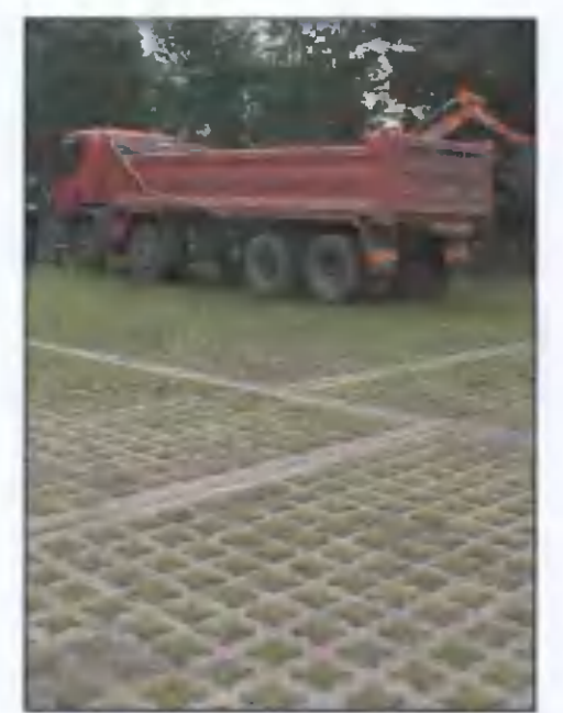
OUTLINE OF AREA OF REINFORCED GRASSCRETE TO FACILITATE TURNING OF FIRE TENDER
