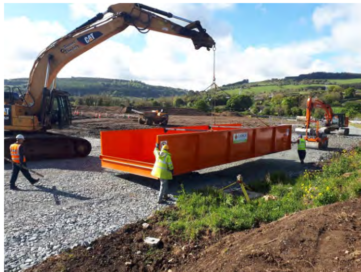
Fig 1 – Wheel being set up on site.
