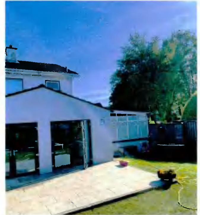
Photo of existing rear elevation
