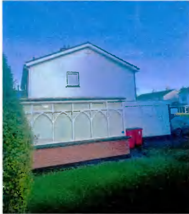
Side view of existing conservatory
