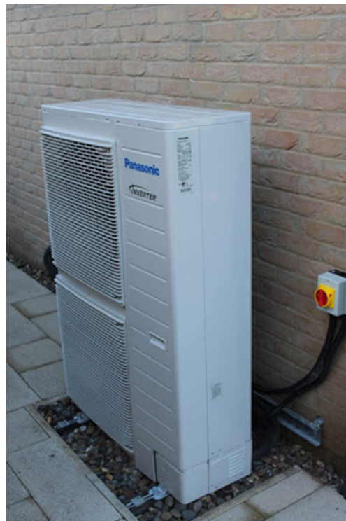
Fig. 4.4 – Typical Air Source Heat Pump Installation
