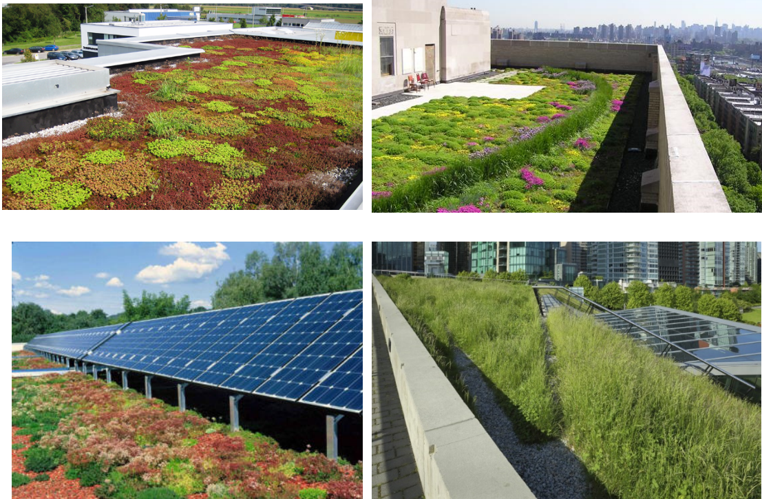
Figure 9.1 Blue Roof Solutions
