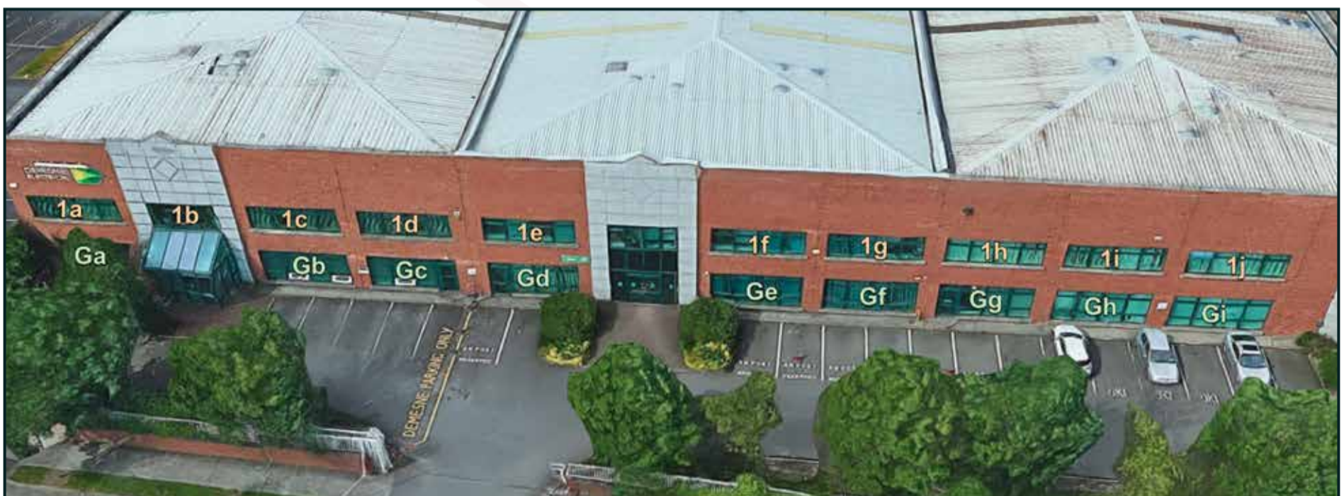
Figure 6.5: Top - Highlighted areas indicate the position of assessed windows., Right - Aerial view of assessed location
