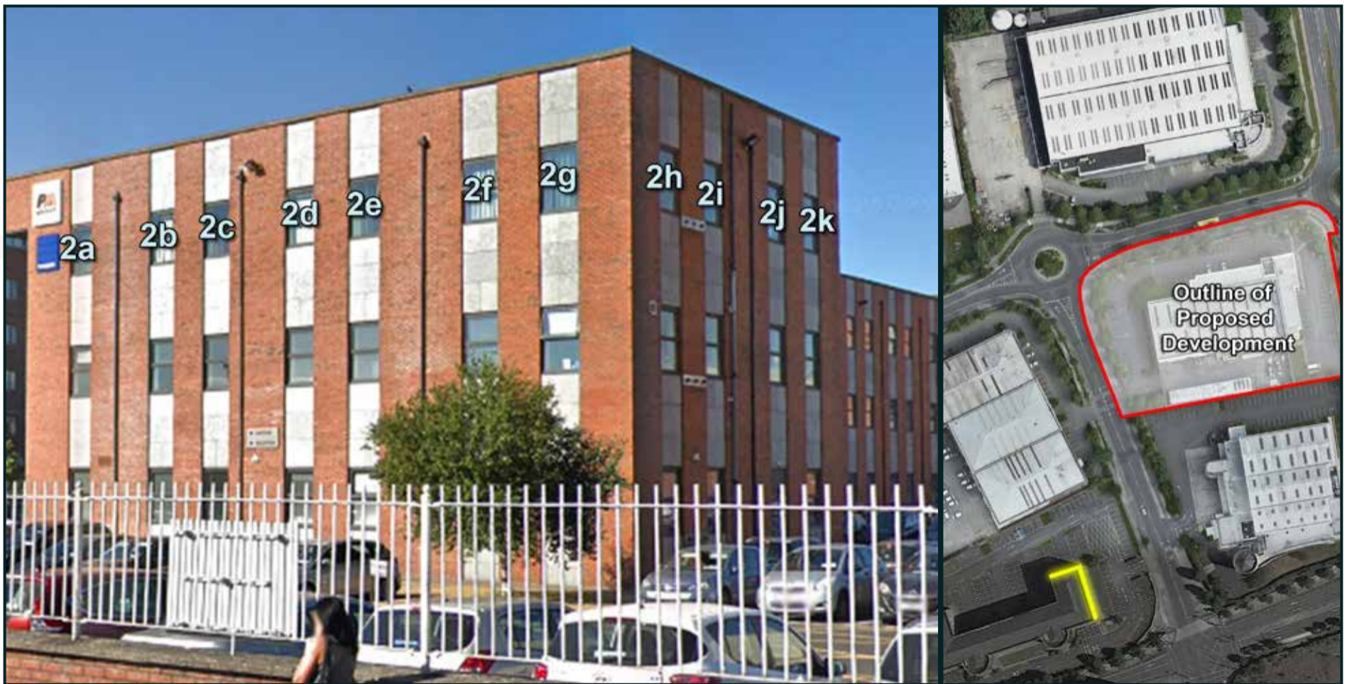
Figure 6.4: Left - Highlighted areas indicate the position of assessed windows., Right - Aerial view of assessed location
