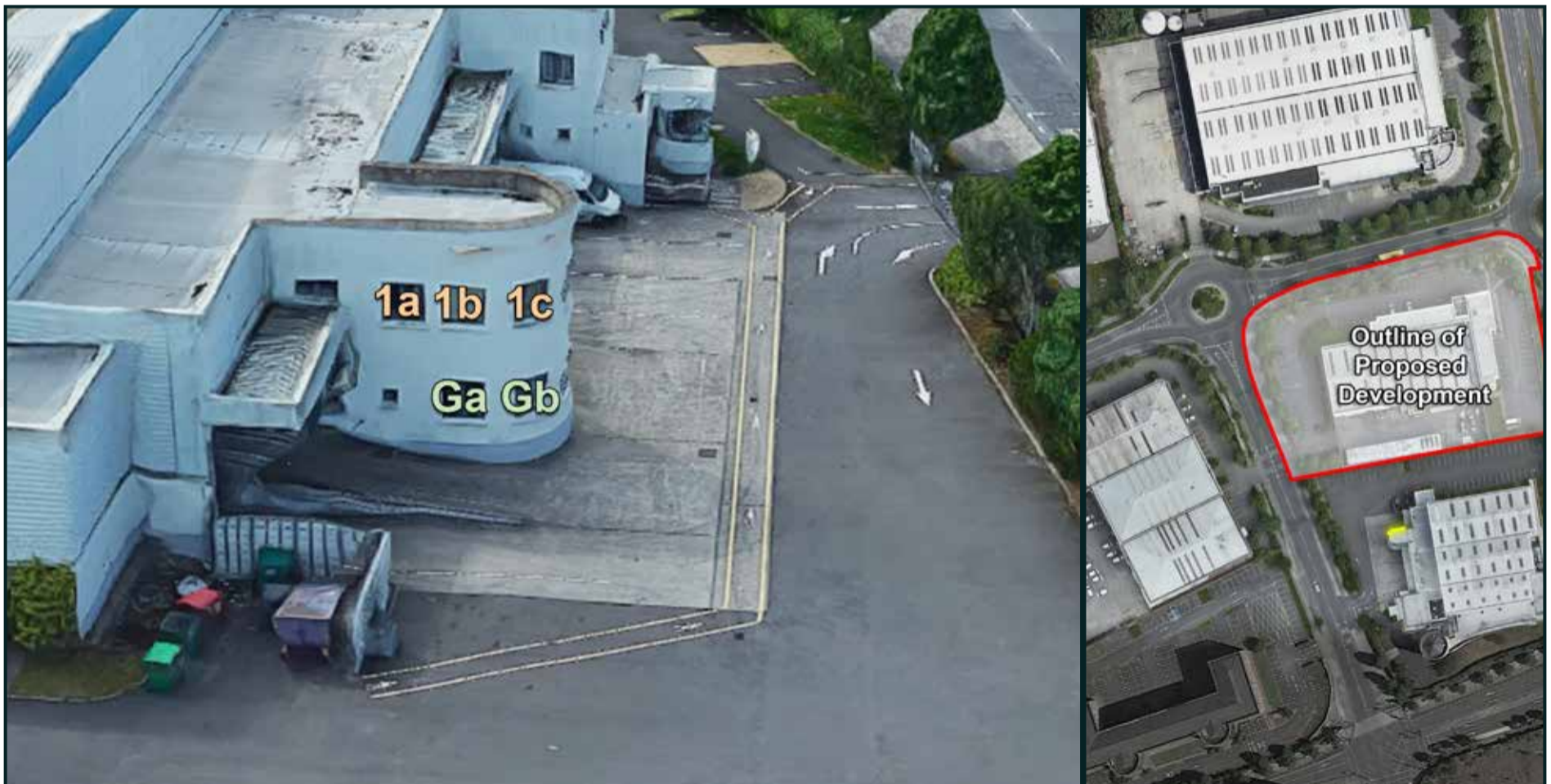
Figure 6.1: Left - Highlighted areas indicate the position of assessed windows., Right - Aerial view of assessed location
