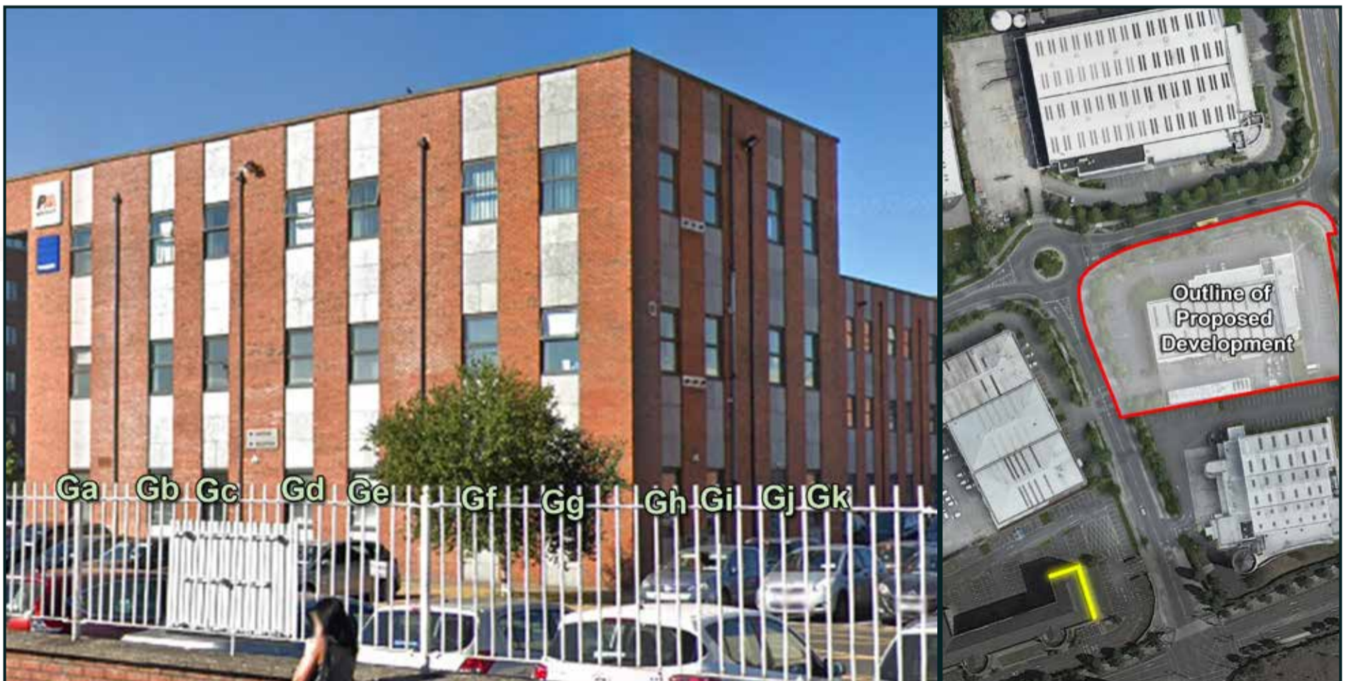
Figure 6.2: Left - Highlighted areas indicate the position of assessed windows., Right - Aerial view of assessed location
