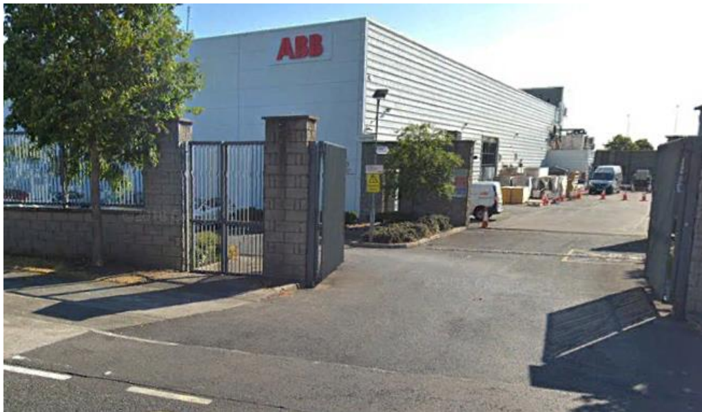
Plate 3: Proposed development area, facing east (Google Street View)
