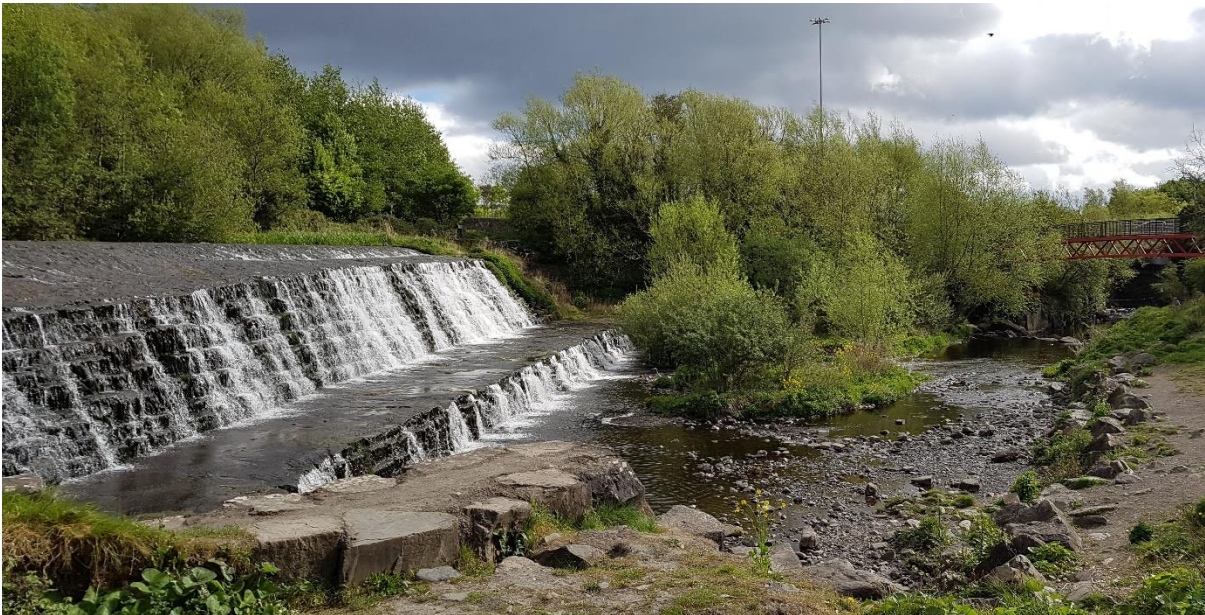
Figure 6.4: the Dodder Weir (Source: Google Images, 2021).
