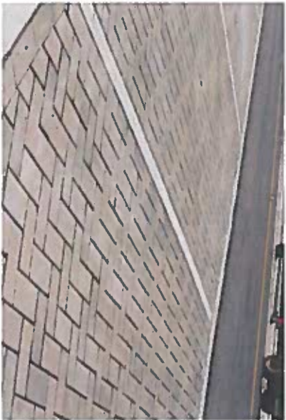
Rustic Paving Block to on street parking
