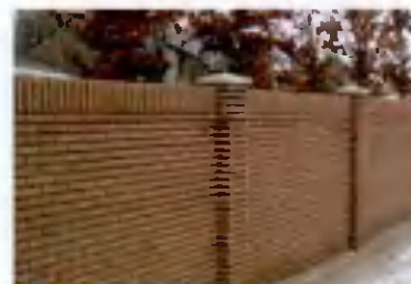
Brick Wall (planting to soften in front)
