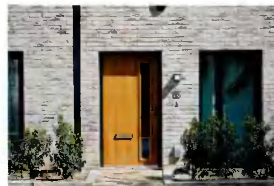
Dark window and door frames
