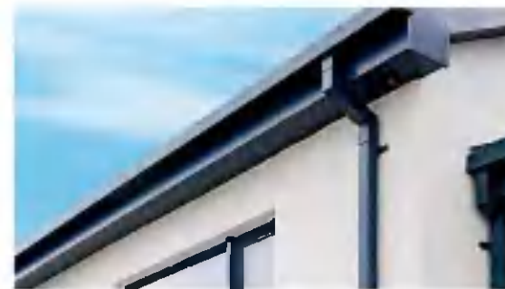
Dark guttering and downpipes
