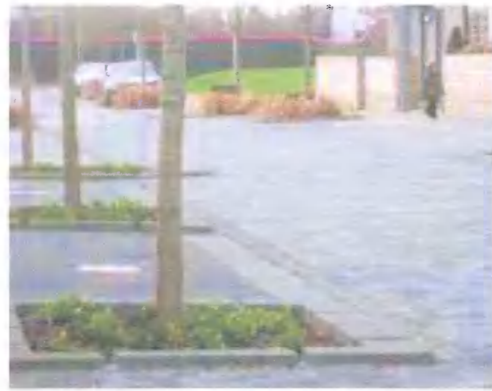
FIGURE 19.16: EXAMPLE OF INLETS TO ALLOW SURFACE WATER RUNOFF TO INFILTRATE INTO TREE PITTS. TAKEN FROM CIRIA REPORT C753 THE SUDS MANUAL.
