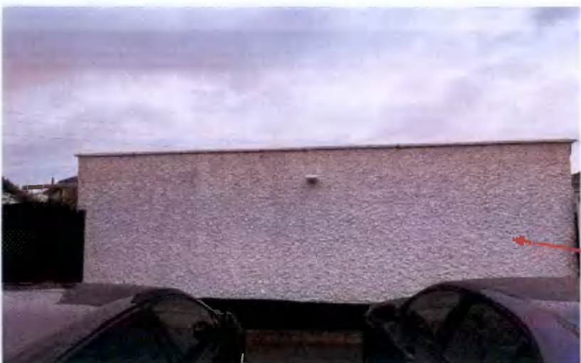
Rear elevation of existing garage for demolition.
