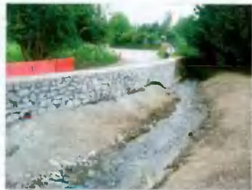
Figure A4 After Wall Reinstatement 2008
