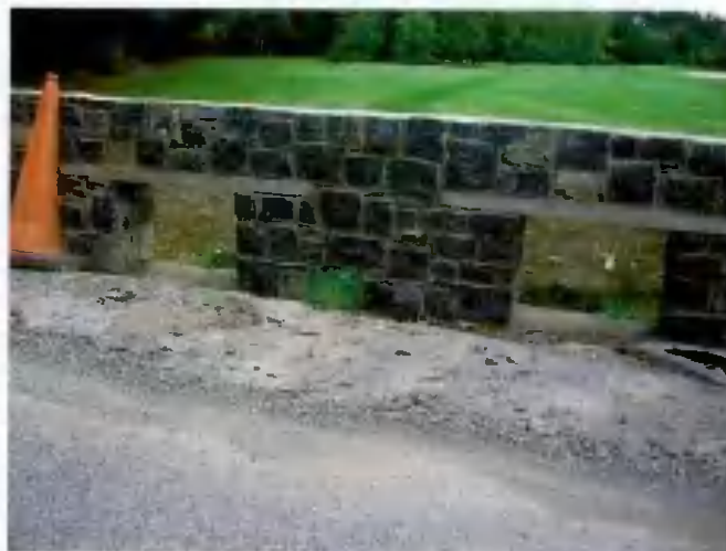
Figure A5 New Opes After Wall Reinstatement 2010
