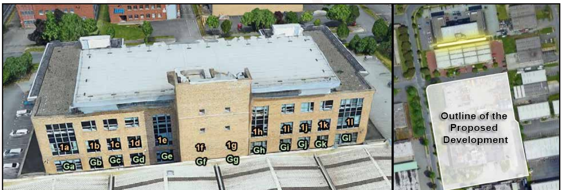
Figure 5.1: Left - Highlighted areas indicate the position of assessed windows., Right - Aerial view of assessed location
