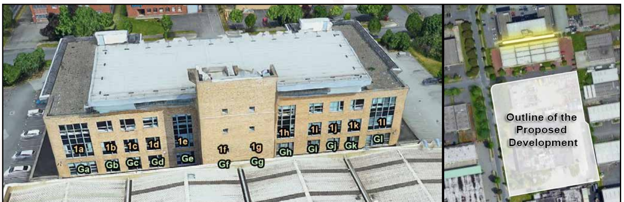
Figure 5.7: Left - Highlighted areas indicate the position of assessed windows, Right - Aerial view of assessed location.
