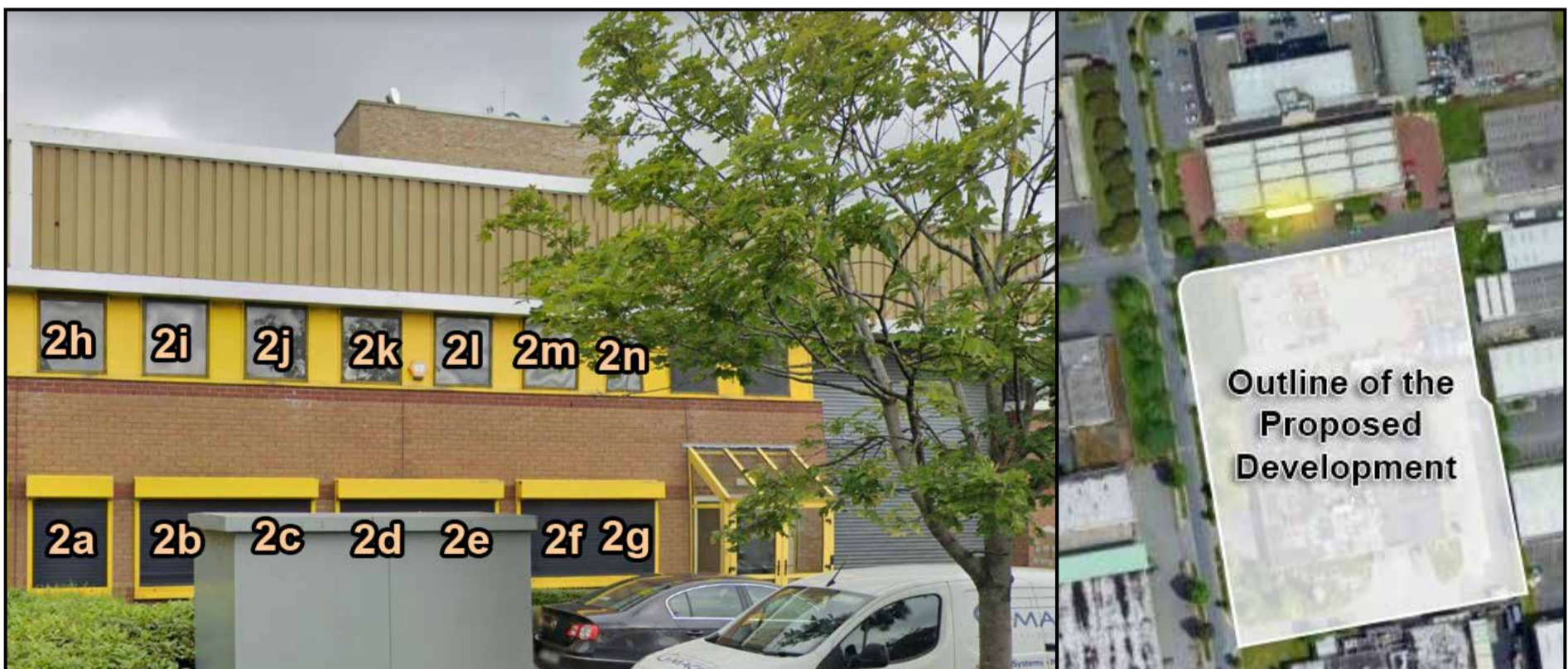
Figure 5.4: Left - Highlighted areas indicate the position of assessed windows., Right - Aerial view of assessed location
