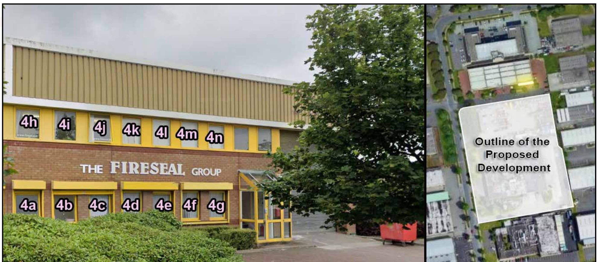
Figure 5.18: Left - Highlighted areas indicate the position of assessed windows, Right - Aerial view of assessed location.
