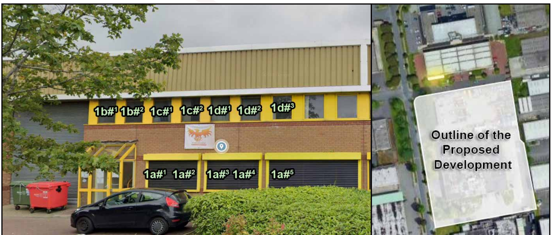
Figure 5.3: Left - Highlighted areas indicate the position of assessed windows., Right - Aerial view of assessed location
