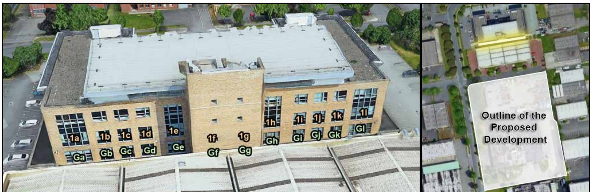
Figure 5.8: Left - Highlighted areas indicate the position of assessed windows, Right - Aerial view of assessed location.
