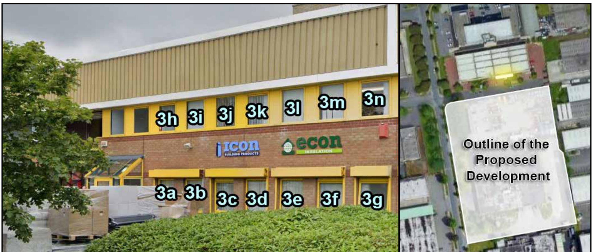
Figure 5.5: Left - Highlighted areas indicate the position of assessed windows., Right - Aerial view of assessed location
