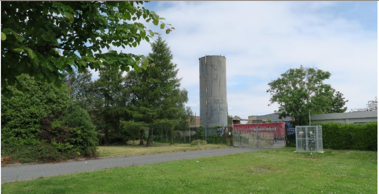
View from Broomhill Road towards southern part of Application Site including the 12m high tank that serves as a local landmark in the townscape
