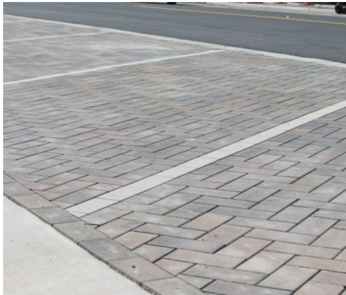
Parking Bays Precast Concrete Permeable Paving
