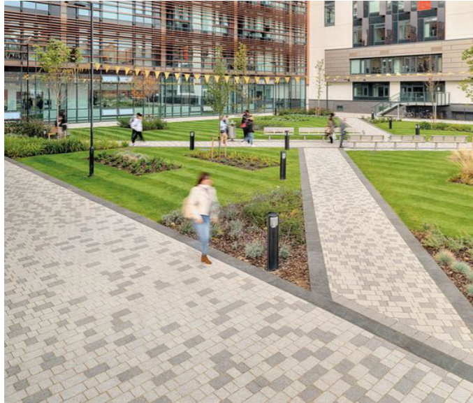
Pedestrian Access Precast Concrete Permeable Paving
