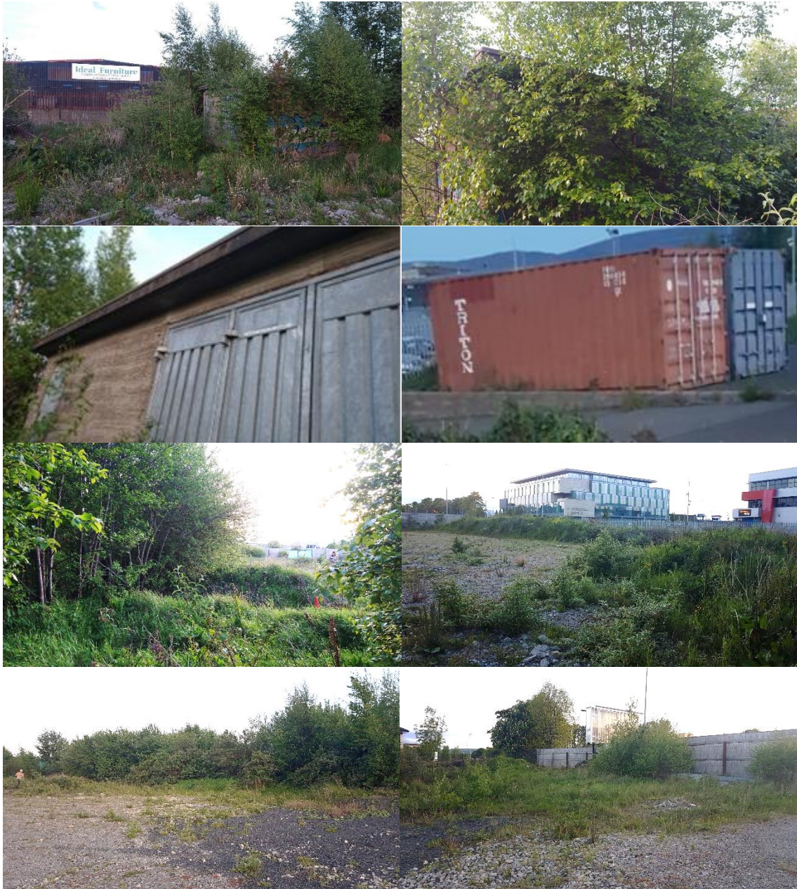
Structures within the site: electricity substation and freight containers and immature tree cover and scrub within the site
