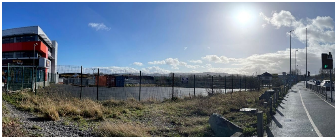
Plate1: Existing site as viewed from Greenhills Road
