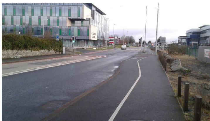
Plate 4 – Existing Greenhills Road /Airton Road Junction
