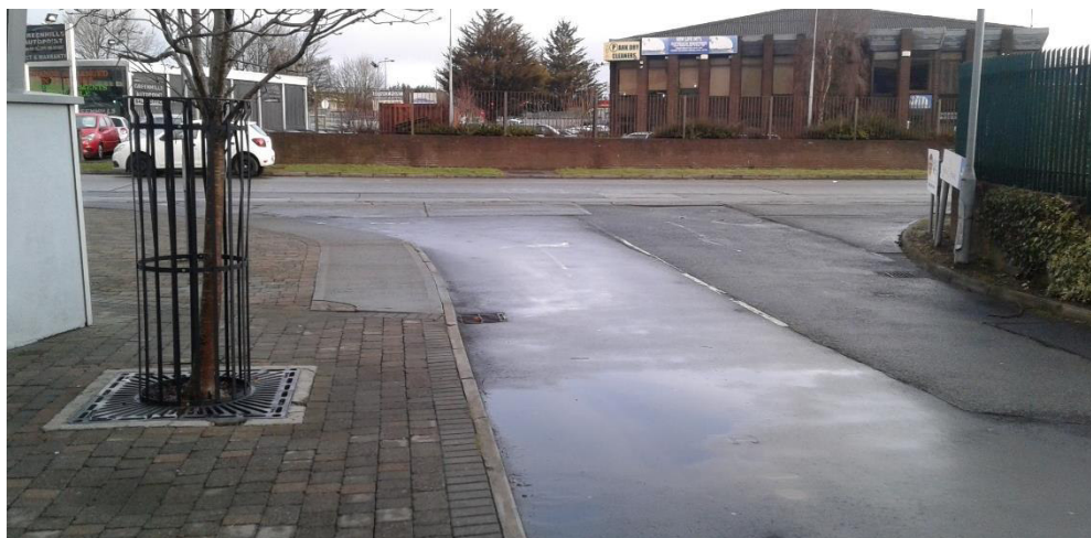
Plate 2 – Existing Hibernian Industrial Estate Road / Development Access Road Junction
