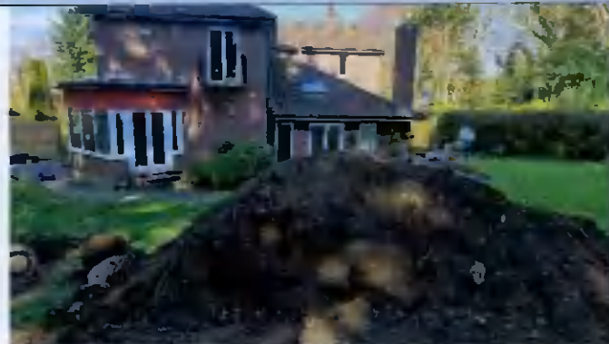
Facing North From the Trial Hole Excavation
