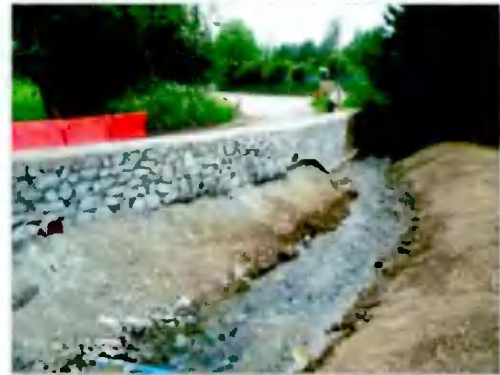
Figure A4 After Wall Reinstatement 2008
