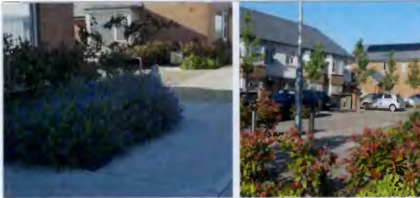
Examples of front boundary planting to public pathway and homezone at Alderke Adamstown.
