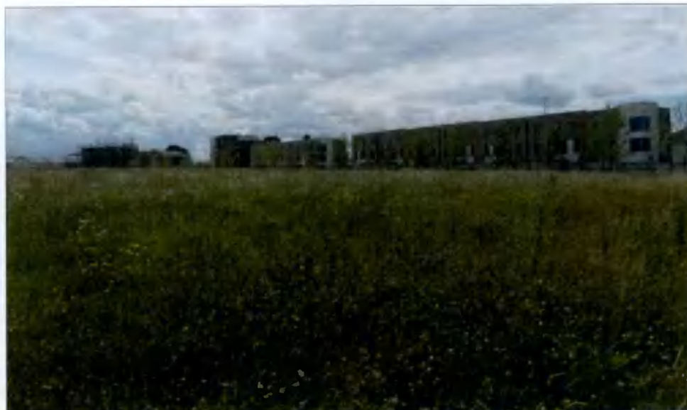
Figure 2.4: Image of the Site Looking West Also Showing Recent Development within the Tobermaclugg Development Area (Development Area No. 4).
