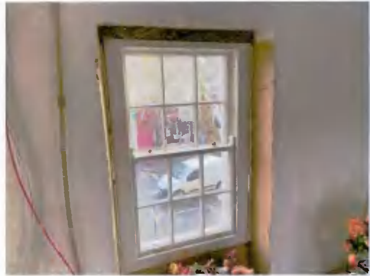
No. 31 First floor - First Floor New hardwood replacement sash window retained to front
