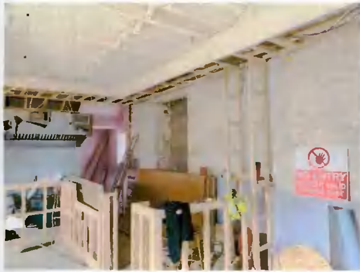
No 23.1 Ground Floor - view towards new servery rear wall area
