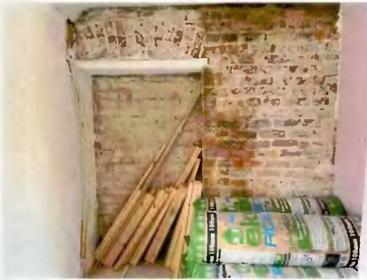
No. 27 First floor - View of gable wall to end gable at rear
