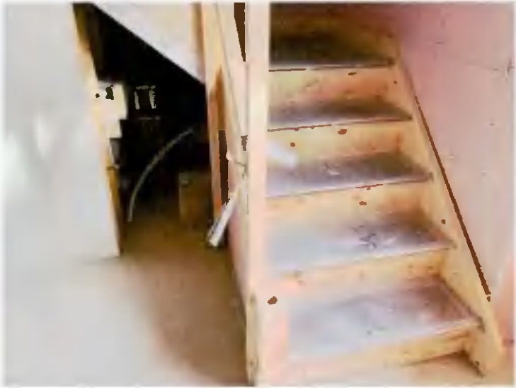
No 24 Ground Floor - View of existing modern stairs to be removed
