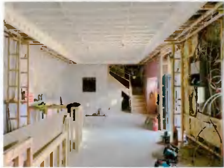
No 24.1 Ground Floor - view towards ex stairs and toilet area
