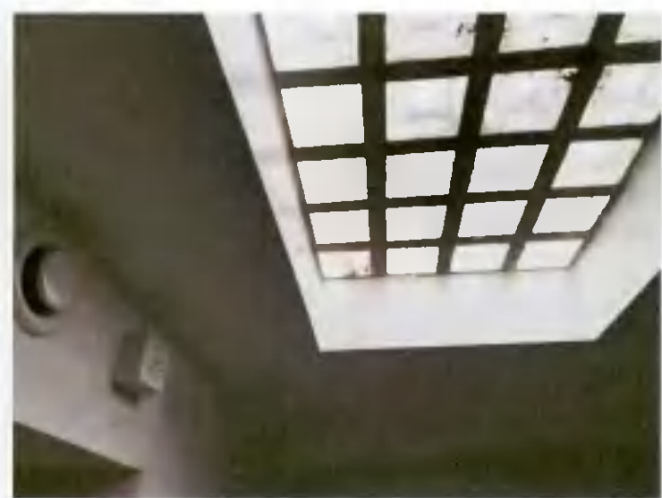
No. 15 Basement Apartment - glass block lay light from bathroom
