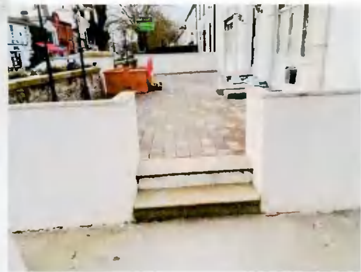
No 5 Existing Front Courtyard Garden with new stone steps from side
