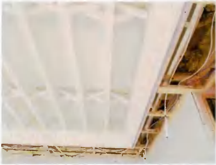
No 22 Ground Floor - Ceiling Detail showing original firsty floor retained
