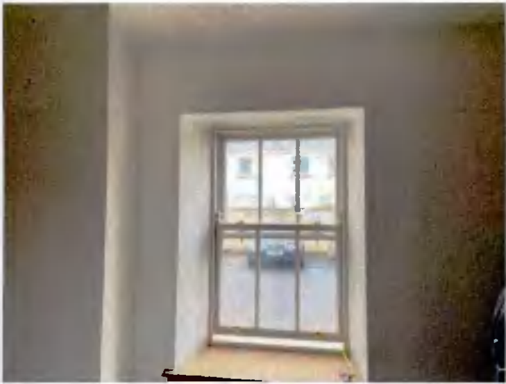
No 17 Basement Apartment - new hardwood window to replace old uPVC
