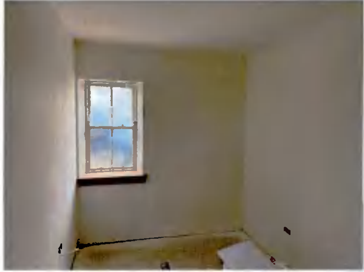
No 20 Basement Apartment Bedroom no. 2 - replacement window
