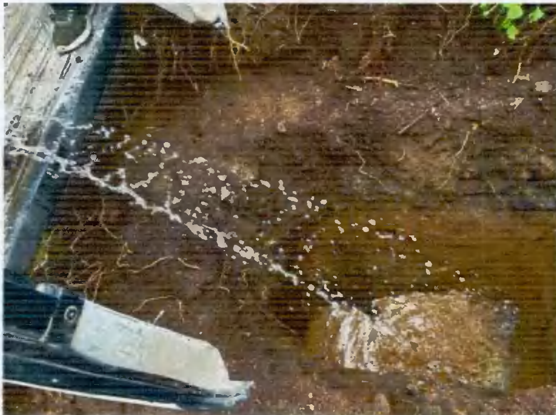
Figure 1.5. Pic showing water discharging quickly into trial pit
