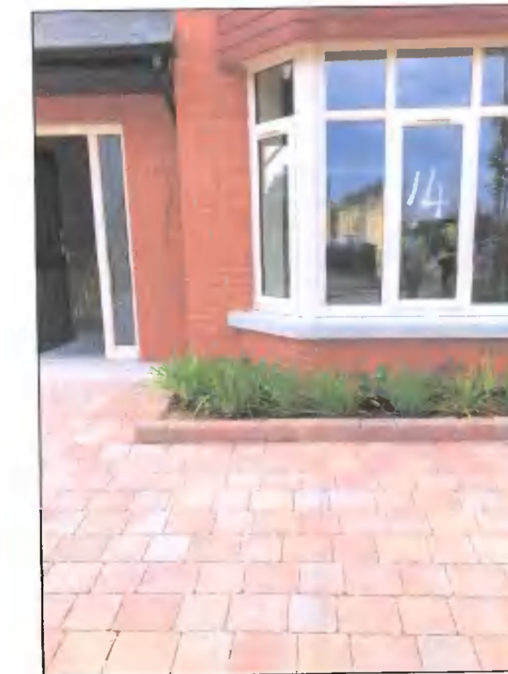
TYPICAL VIEW OF PERMEABLE PAVING
