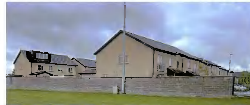
Block work wall edge to existing neighbourhood to the south-east and existing gates to facilitate future access to and from Silken Park Avenue
