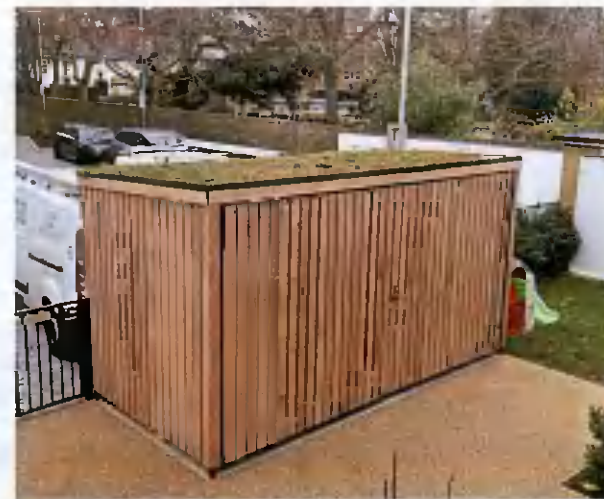
Bike store with sedum green roof
