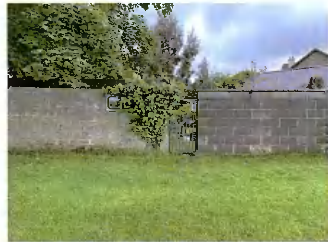
Rear wall of residential property to west
