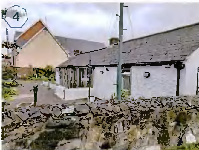
Single-storey house along Naas Road, with stone walls and sloping roof
