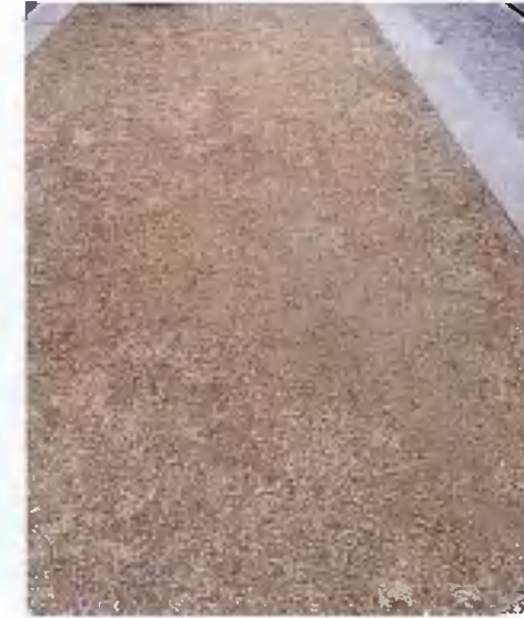
Rolled gravel / dust paving.
