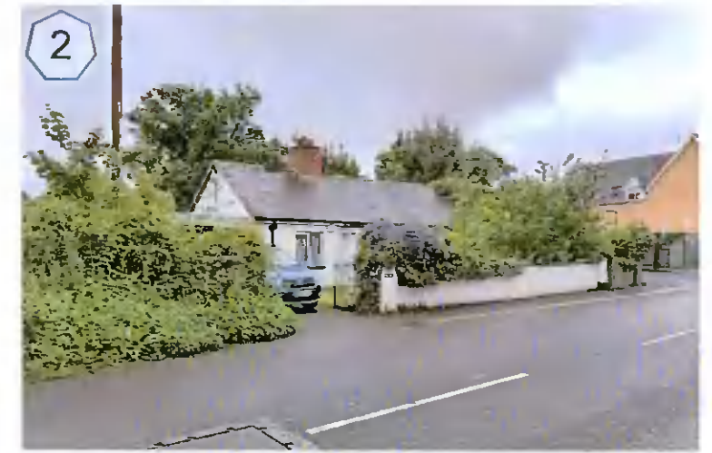
Single-storey one-off dwelling to western corner of the site along Old Naas Road
