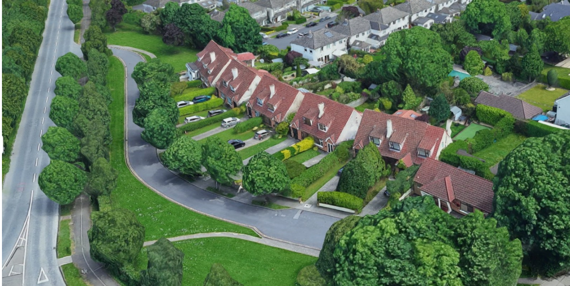
Image 1 : Aerial view of Templeroan Lodge, note steep pitched dormer bungalows.
