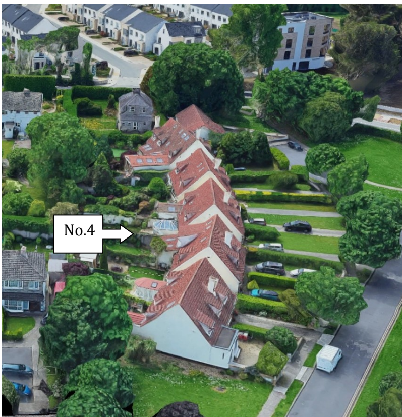
Image 2 : Aerial view of Templeroan Lodge, note simple first floor dormer rear extension ( No. 4 Templeroan Lodge) designed in keeping with the original dwelling.
