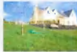
▶ Very low visual impact from fully installed units.
