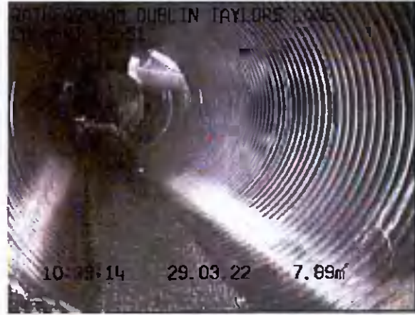
CULVERTX_6f57a131-da16-41a9-9b17-a8bc14d7d968_2022 0329_104149_390.jpg, 00:01:19, 7.89 m Pipe material changes to polypropylene at this point
