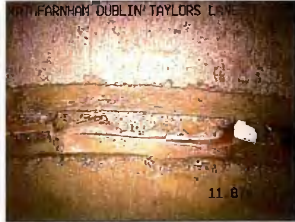
S6X_e184c169-363a-4da8-88e6-14cf39badc3a_20220330_12 4638_960.jpg, 00:02:19, 11.87 m Open joint, large
