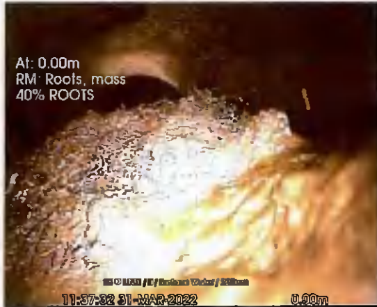
S5 US LINE1_0-00m_113732.jpg, 00:00:02, 0.00 m Roots, mass, 40% cross-sectional area loss, ROOTS
