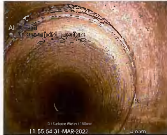
G2 DS S4_4-65m_115554.jpg, 00:00:26, 4.65 m Open joint, medium
