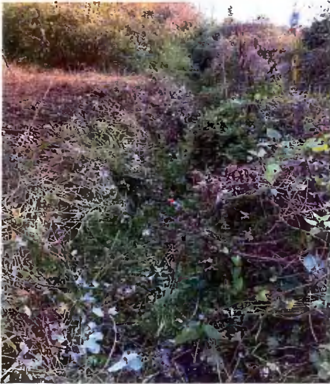
Existing Old Mill Drainage Channel 01
