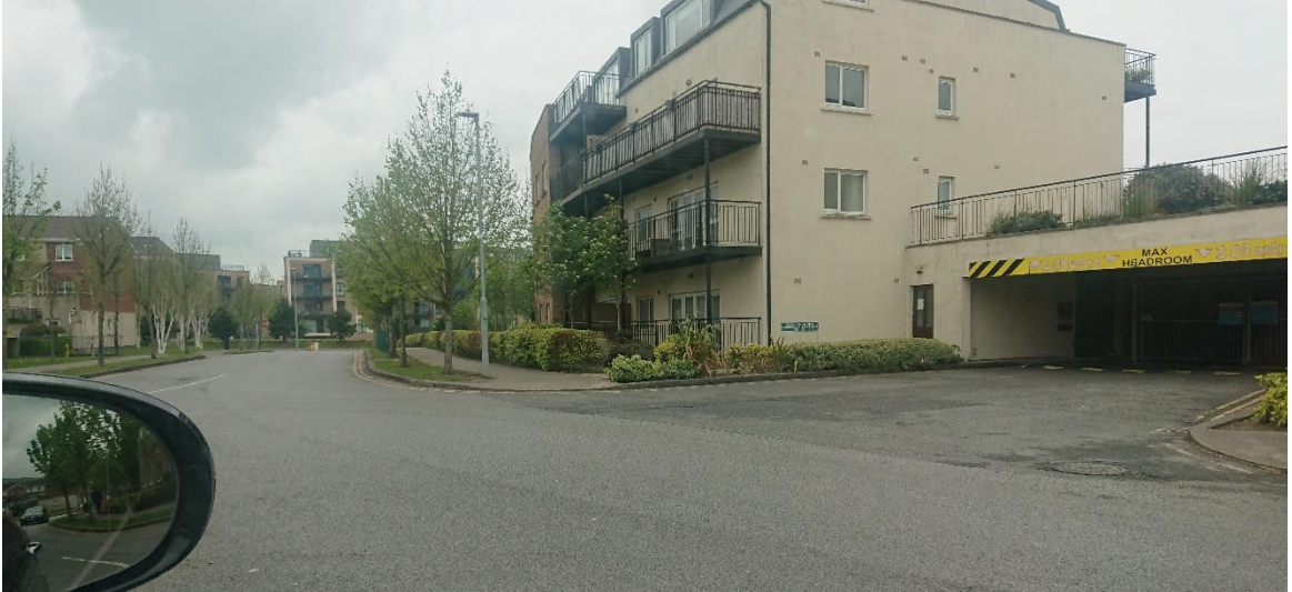
Pic 3b – Same junction taken from the Yield road marking in pic 3a and showing proximity of the Fortunestown lane junction (apartment blocks at end of road)
