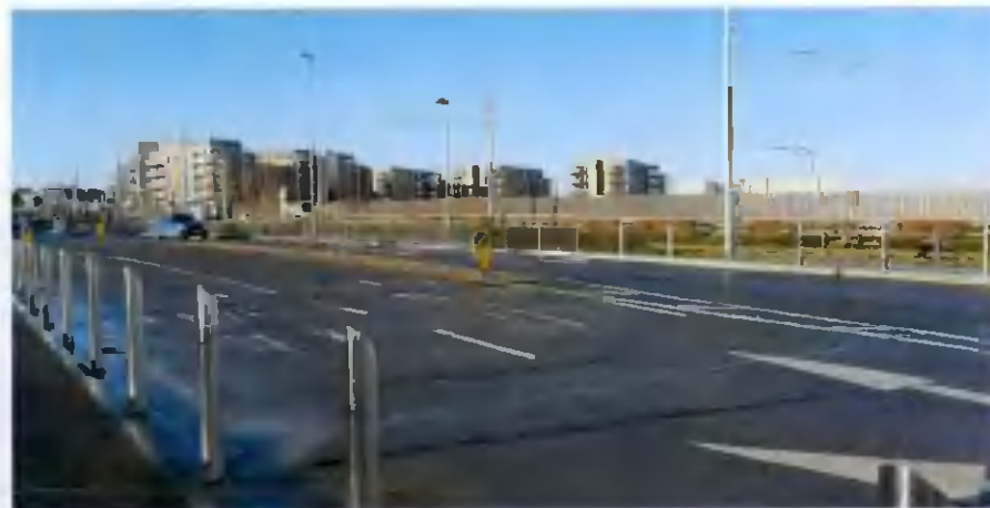
Figure 3 - View of the site from South East - VIEW 1
