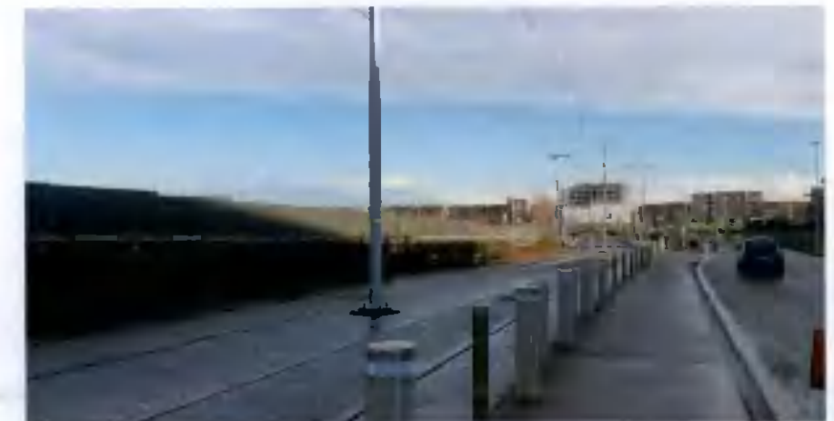
Figure 5 - View of the site looking from South - West - VIEW 3
