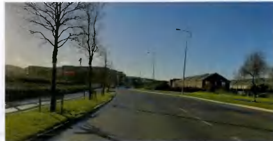
Figure 4 - View of the site looking from north - VIEW 2
