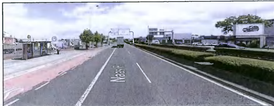
Fig. 2.2 Eastbound view of existing advertising panel from Naas Road
