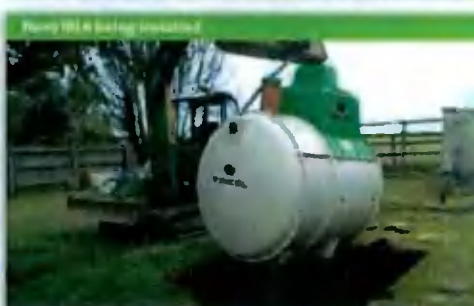
Novo IRL 6 Wastewater treatment plant installed
