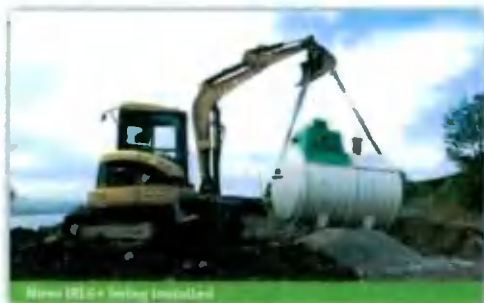
Novo IRL 50 Wastewater treatment plant installed
